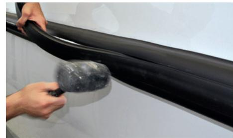
Apply the closing profile by pressing with a rubber hammer.
