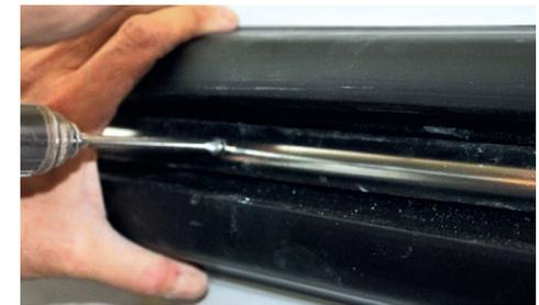
Apply the second base module, then tighten the screws until completely secure the base parts. The modules have to be placed perfectly under the steel track.
