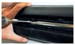
Apply the second base module, then tighten the screws until completely secure the base parts. The modules have to be placed perfectly under the steel track.
