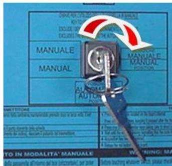
1. Quickly turn the key on the cover from [AUTOMATIC] to [MANUAL], leaving it on [MANUAL] at the third time.
