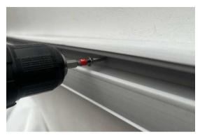
Drill the base with screws to fix it to the boat.
