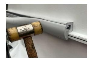
Applying the top profile by pressing with a rubber hammer.
